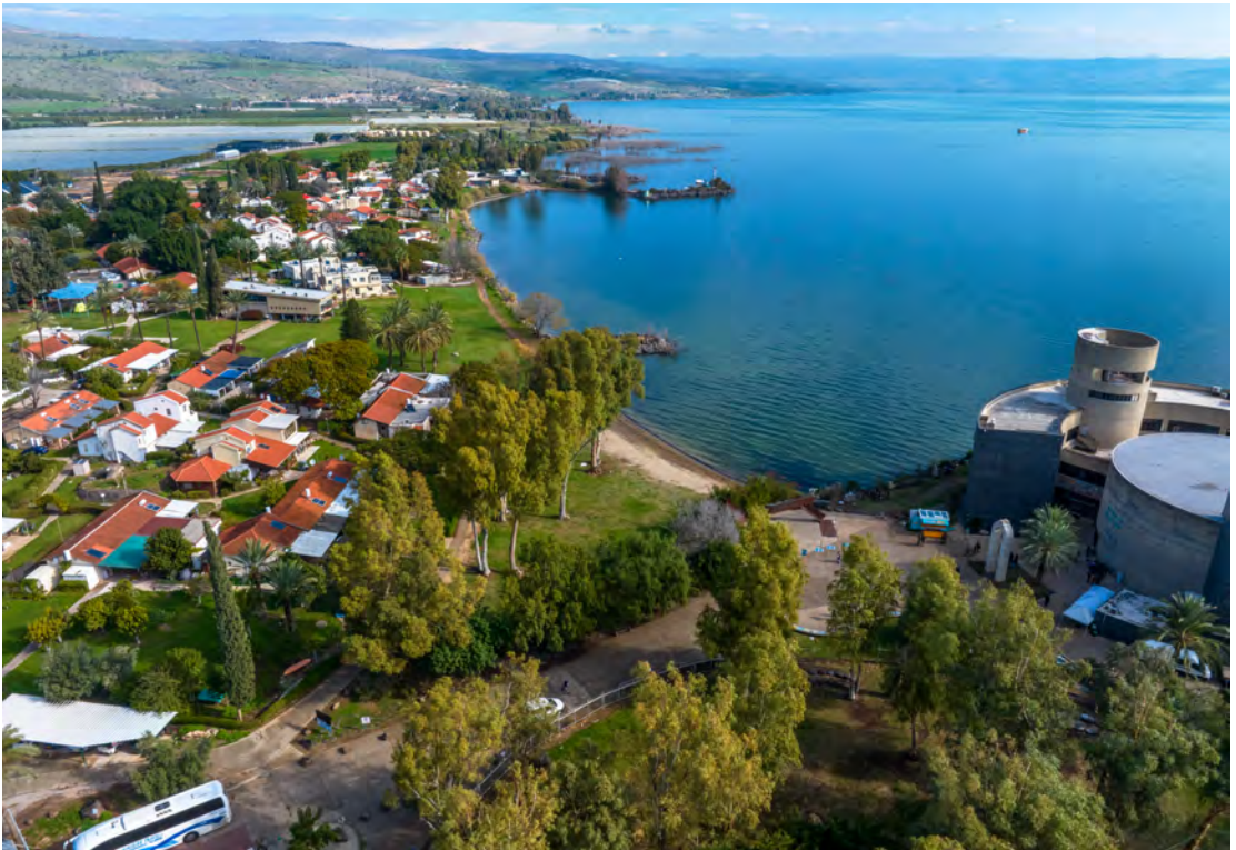
VIEW NORTH: KIBBUTZ GINOSAR ON THE NORTHWEST SHORE OF THE SEA OF GALILEE, WITH THE YIGAL ALLON CENTER (RIGHT). THE FIRST-CENTURY AD GALILEE BOAT WAS DISCOVERED HERE.
